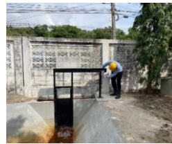
Fig No. 3 Closed rain gutter gate
